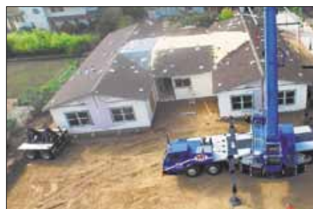
The home comes together.
